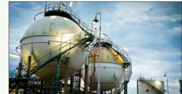
Korea Gas Corporation Substation 21 in Pyeongtaek
